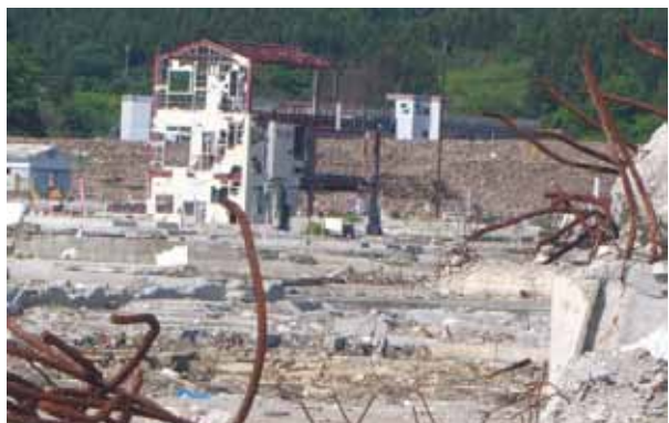
Damage due to the Great East Japan Earthquake and Tsunami
