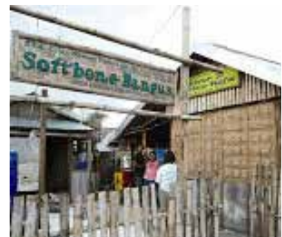
Building for the Marine Products Processing by Women's Group
